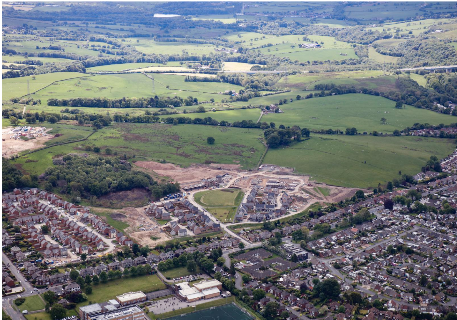
S106 contributions have been received from the new residential development at Gib Lane in Blackburn
